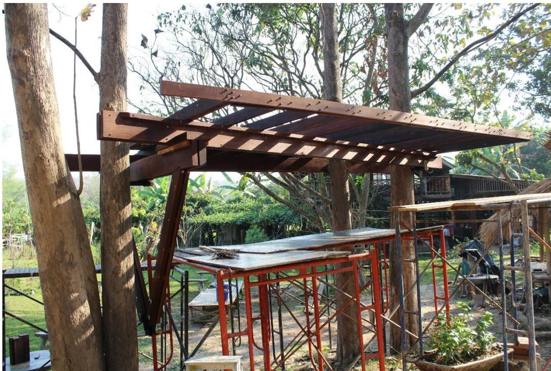
**Fig. 4** Installed floor frame.
