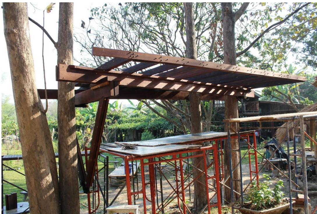
Fig. 4 Installed floor frame.
