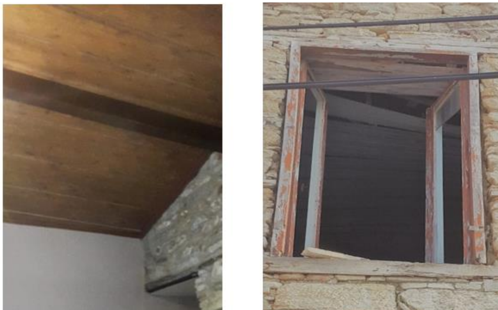
Figure 6. The wooden ceiling and window
