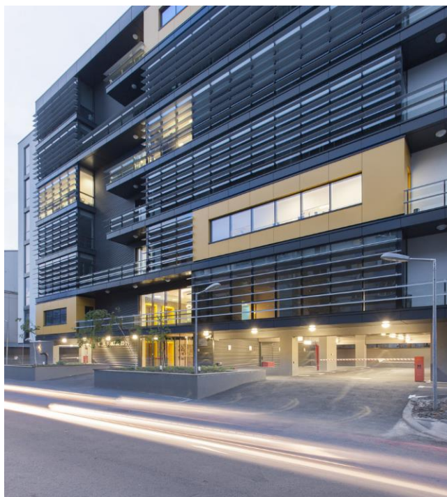
Figure 4: CSDA Siriului. Sun protection system on the South Facade. © Andrei Margulescu, Marius Grigore
